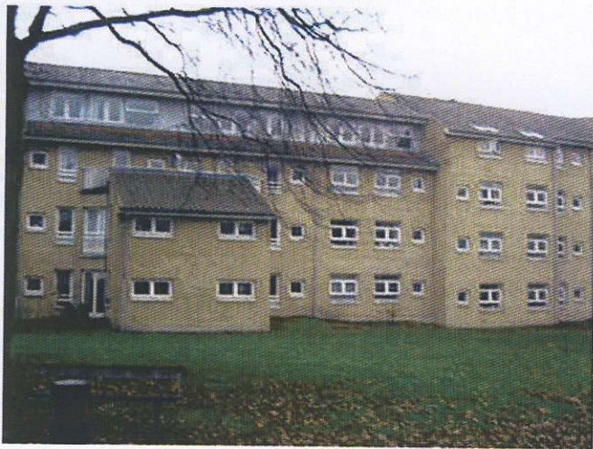
Facade mod have / hav, opgang 1-16
