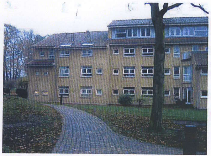
Facade mod have / hav, opgang 1-16
