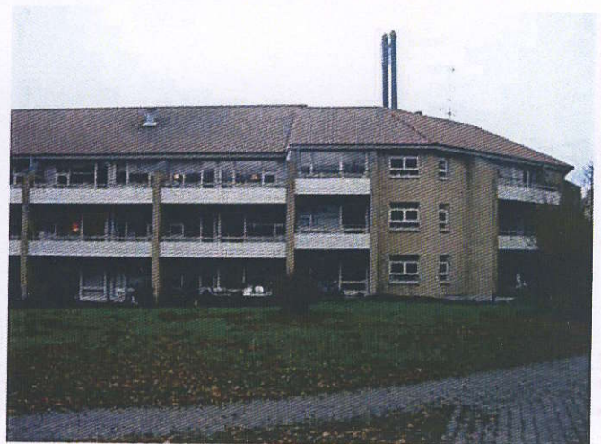
Facade mod have / hav, opgang 1-16
