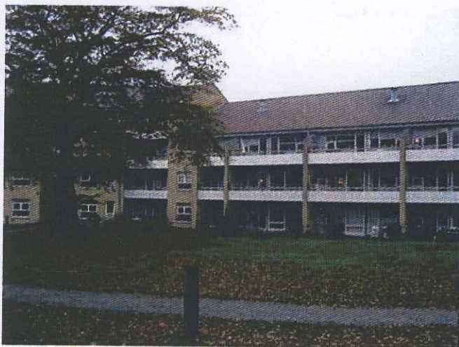
Facade mod have / hav, opgang 1-16
