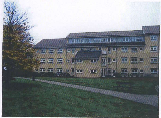
Facade mod have / hav, opgang 17-31
