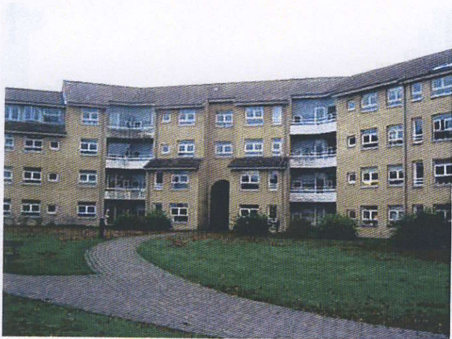
Facade mod have / hav, opgang 17-31
