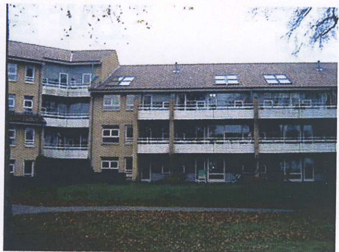
Facade mod have / hav, opgang 17-31
