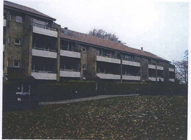
Facade v. opgang 1-4
