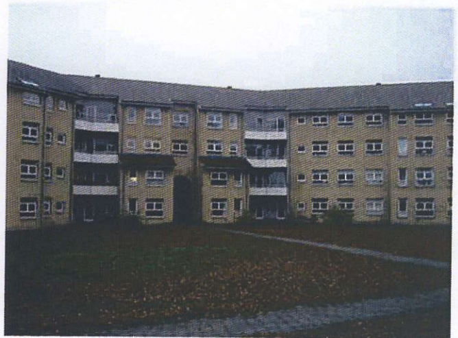
Facade mod have / hav, opgang 1-16
